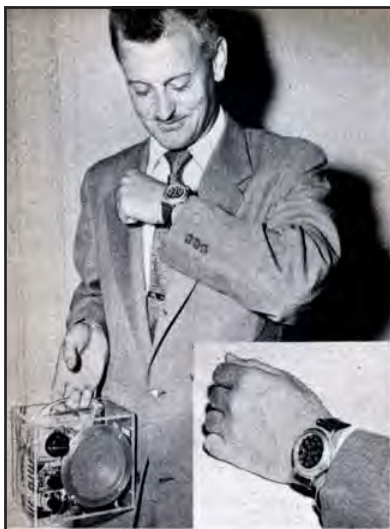
James Sutherland, General Manager of the Electronics Division of Sylvania Electric Products, Inc., hears his voice through transistorized radio receiver while he broadcasts into his wrist radio.
